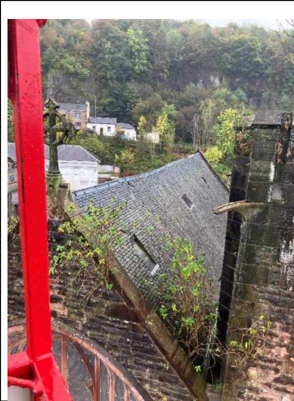
North Elevation Showing Vegetation and Apex Deflection
