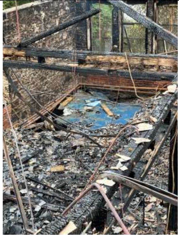
First Floor Collapse in Southeast of North Wing
