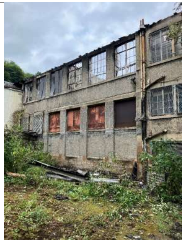
East Elevation of Central Wing
