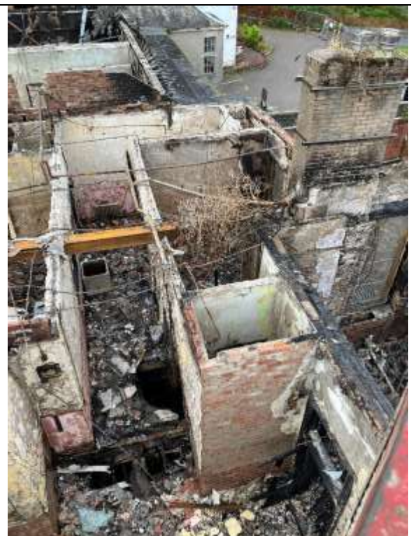
Cellular Walls With Lateral Movement
