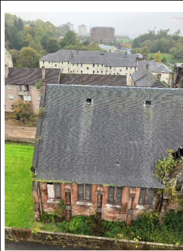
View of Roof
