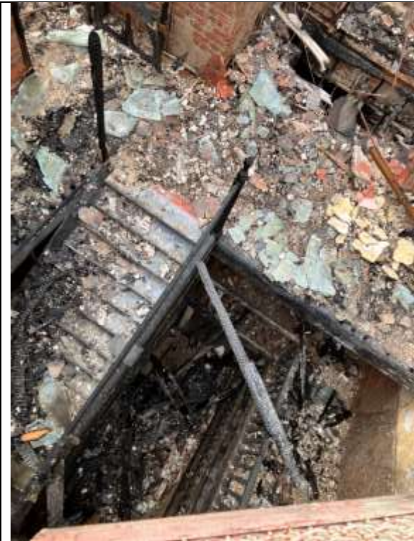
Stair Core from Above
