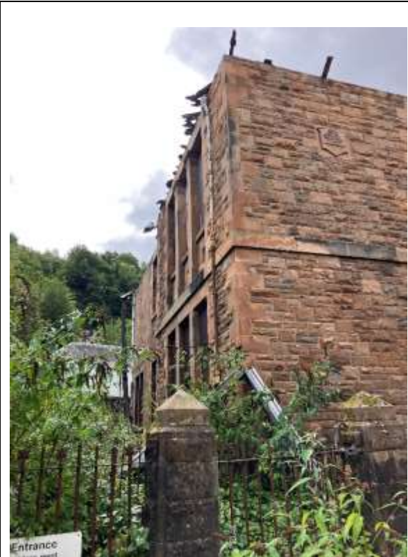
View on Northeast Corner
