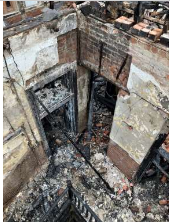
Internal Wall Construction
