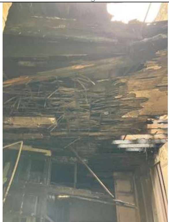
First Floor Collapse in Southeast of North Wing
